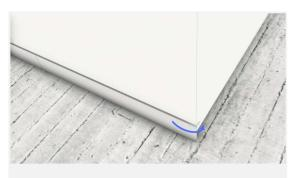
For the next skirting board, also provide a piece of stretched tape at the end. Attach this skirting board over the protruding piece of tape from the previous skirting board.
