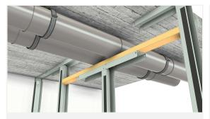
Position timber under the pipes and between the I-modules on the left and right of the central module.
