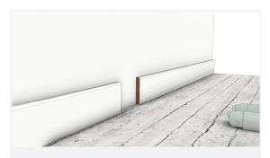
Make a recess in the skirting board the width of the wall.
