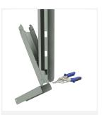
Fold the profile piece over and cut the bottom edge.
