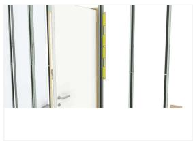
Hang the door leaf. Level the C-module on the hinge side.
