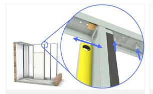
Level and fix the top of this C-module. Put a wooden block between the C-module and the door profile if there is too much play.
