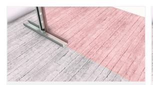
Centre the horizontal and vertical profile on the laser. Fix this module.
